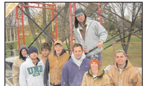
The team, from left to right: Jason Anders, Matt Mulcahy, Alex Raway, Sam Billmeier, Bill Sagissor, DCTC Concrete Masonry instructor Paul Geisler, TJ Lawrence, and Blake Winchell.
