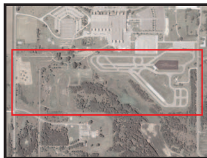
DCTC currently rents the land inside the red box from the University of Minnesota and wishes to acquire it through a bonding bill that is being reviewed this legislative session.
